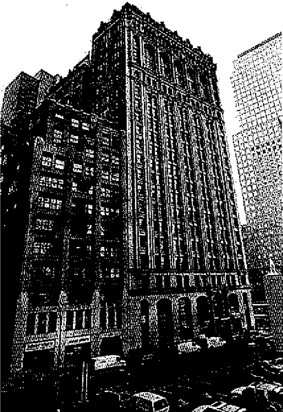
Thornton Tomasetti assessed the physical condition of the 90 West Street building, damaged as a result of the collapse of the World Trade Center, and developed an appropriate course of action to minimize future building deterioration.
